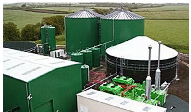
From top to bottom: auto-sorter from a Material Recycling Facility, an autoclave unit and an anaerobic digestion plant.
